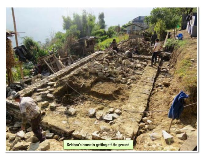
The corner stones from old shelter were all useless so two mason leaders had to work continuously for 10 days to cut the corner stone. Almost 30% of the stone required for the wall was salvaged from the old house. But the wood from the old house was totally unusable.
